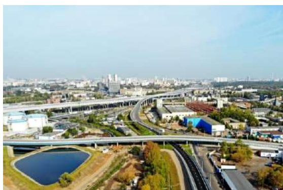
Figure 3. North East Chord of Moscow ( stroi.mos.ru )
